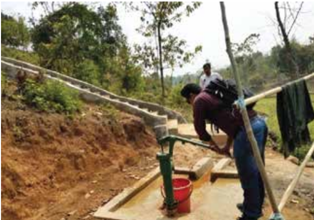
Figure 38: Installation DSTW & Stair at Antu para, Ramgarh.
