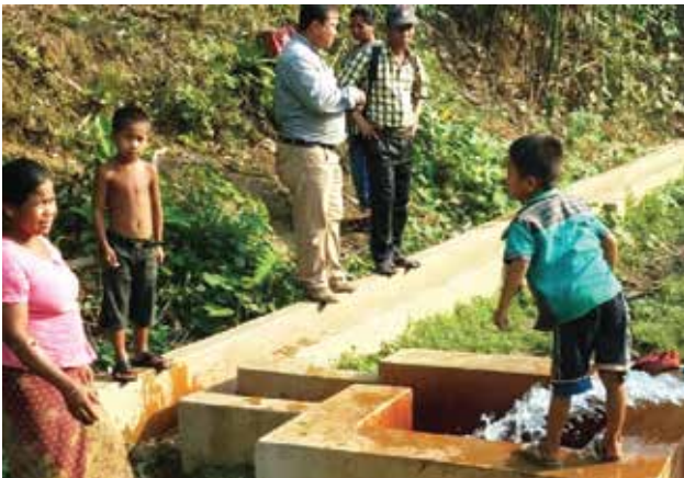
Figure 39: Installation Deep set Tube well for Irrigation at Gabamara Para
