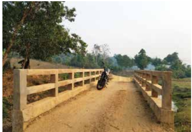
Figure 37: Box culvert at Chailakarbari Para at Laxmichari
