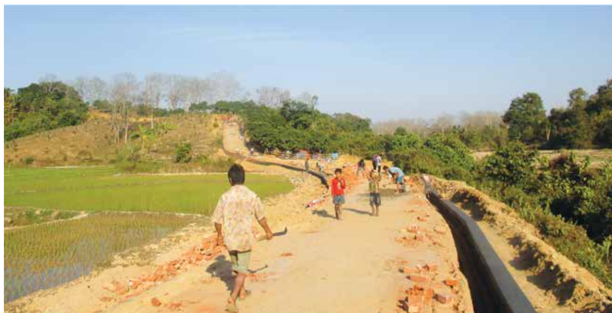
Figure 11 HBB village access road Dharmagar to Dharmapur
