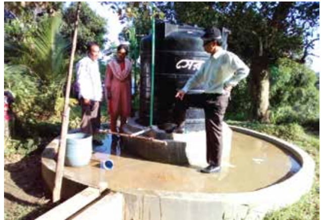
Figure 35: Construction of Water Tank at Uttar Mahalchara Para, Sadar Upazila
