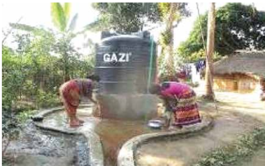
Figure 32 Water reserver at School para in Khagrachari Sadar Upazila
