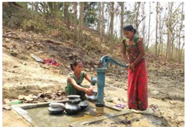
Figure 45: Shallow Tube well Installation at Durung Para, Mahalchari, Khagrachari
