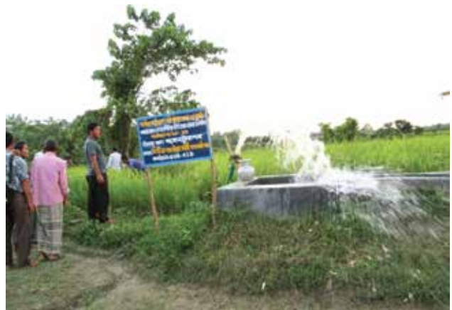
Figure 36: Irrigation for Power pump at Pedia Para, Khagrachari Sadar
