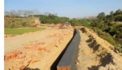
road construction including drainage structures.; (ii) 950.00m of surface(L) drain; (iii) 4 Nos. (U-drain) and 1 No. Culvert; (iv) 192.00m of guide wall. Total budget is BDT-19,881,600/=.
