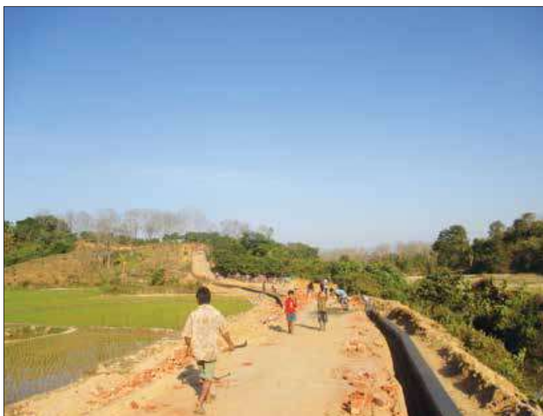
Figure 7 HBB village access road Dharmagar to Dharmapur
