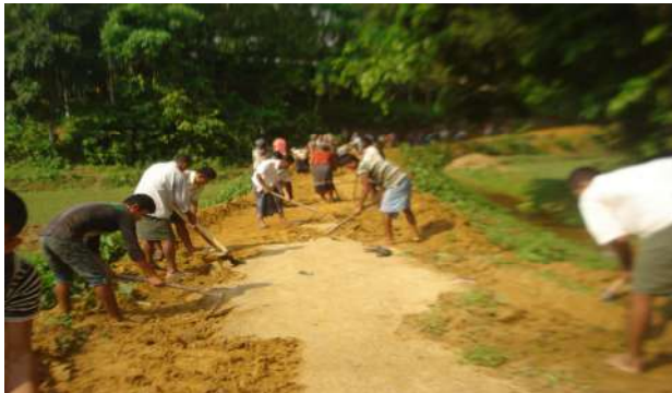
Figure 13: The LCS team members worked at Dharmapur village access road
