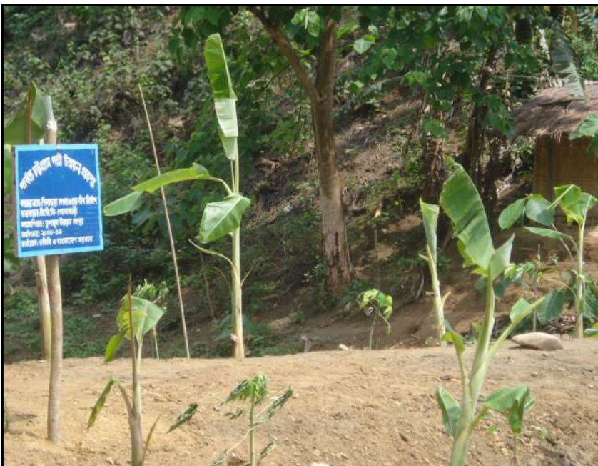
This fish culture dam, built with TUS support, provides infrastructure to help communities improve their livelihoods
