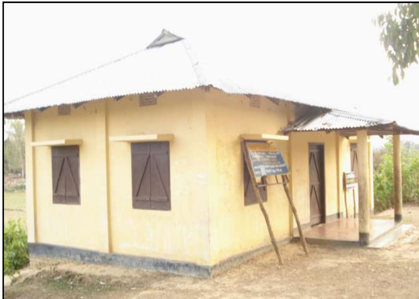
Upper Perachara Literacy Centre, constructed with TUS support, provides space for community education and gatherings
