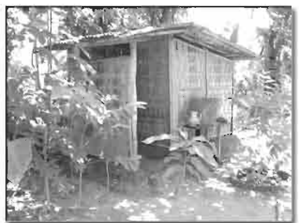
Hygienic latrine Installed by TUS, Baibonchara Union
